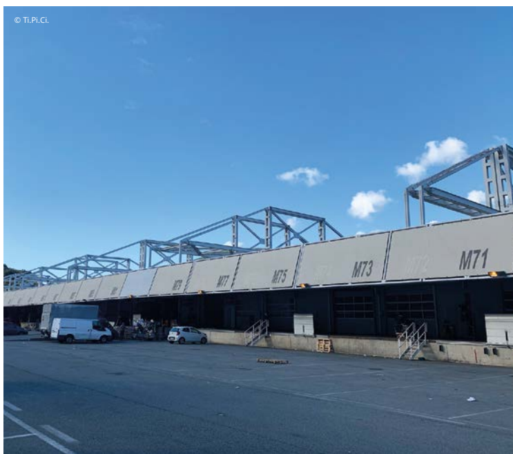
Figures 1 and 2 – The market’s central area is a free space, as there are no supporting pillars.
