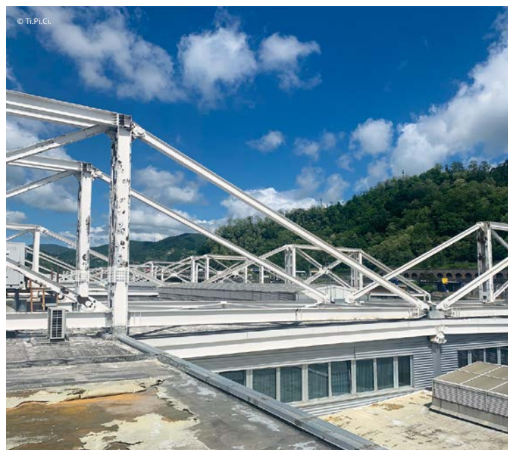
Figures 1 and 2 – The market’s central area is a free space, as there are no supporting pillars.
