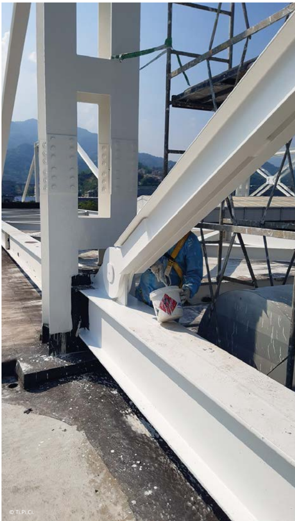
Figure 9 - All water-based paints were applied by brush and roller.
