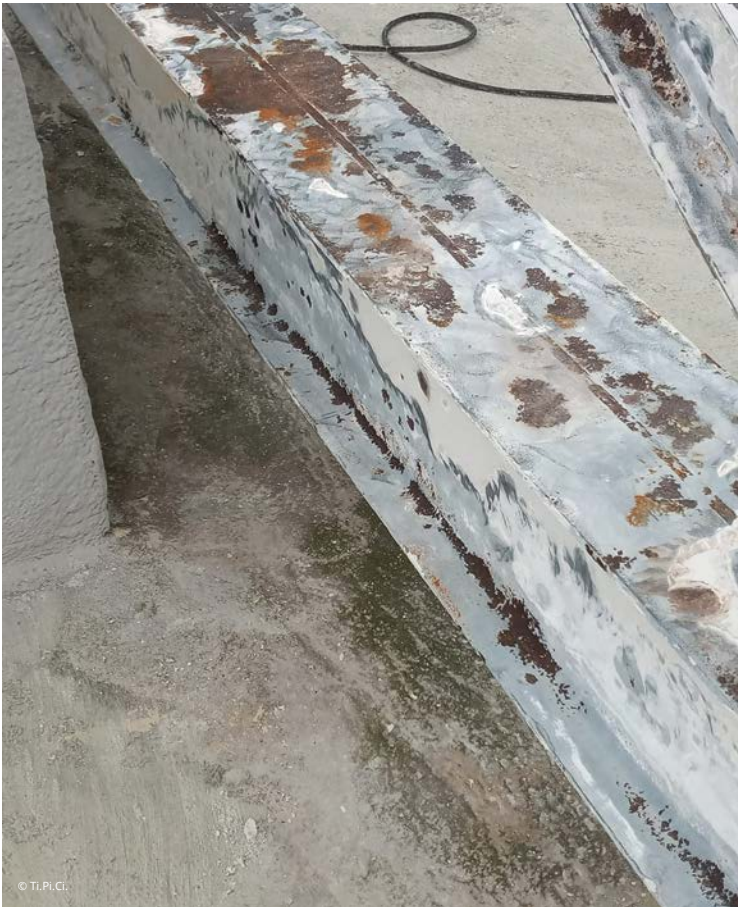
Figures 7 and 8 – Rust was removed by power tool cleaning.
