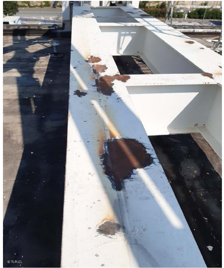
Figures 7 and 8 – Rust was removed by power tool cleaning.
