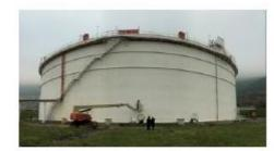
conditions were not very favourable, with strong winds repeatedly interrupting the application. The safety of the operators working at height had to be safeguarded at all costs. Moreover, the air and surface temperature was only 6°C. Despite these low temperatures, the paint was applied equally and without any drying or film hardening problems.
